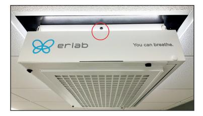
This orifice allows the vacuum downstream of the particulate filter to be monitored. Remove the black plug and measure the relative pressure at the orifice with a suitable pressure gauge.
